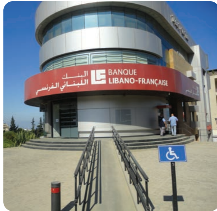
Hazmieh branch equipped with a ramp.
